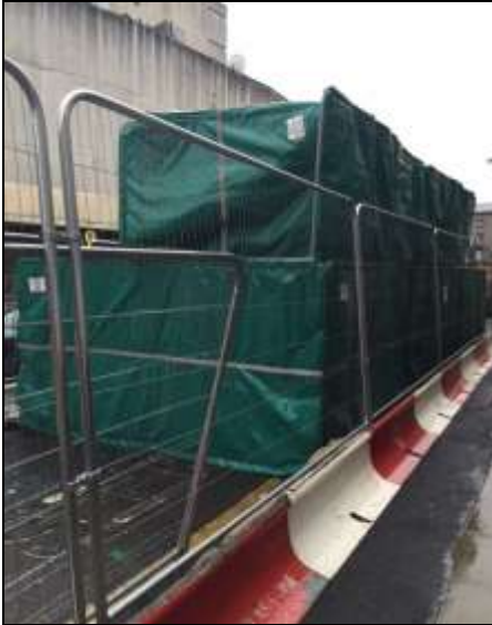
Double height acoustic blanket enclosure
