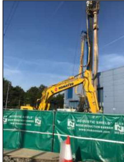
Acoustic blankets screening piling and excavations
